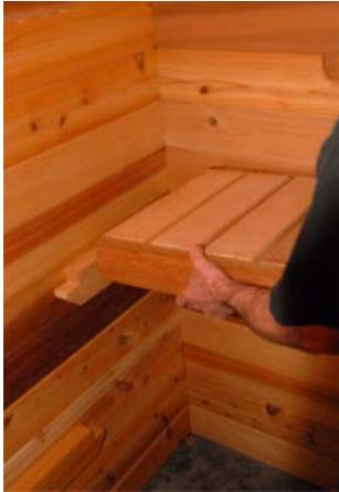
**Step 8:** Wall bench brackets are screwed to the wall with 3" screws and benches are pre-built. With the appropriately labeled bench, insert one end on top of the first bracket with the opposite end at a higher elevation. Once the first end is in place drop the opposite end down onto the bracket. If it is a tight fit, use the rubber mallet to drop in place.
