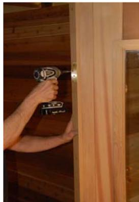
Step 6: Once in place, and the door is plumb, fasten the door/ door jamb to the wall with supplied screws THROUGH THE HINGE MOUNTING HOLES.
