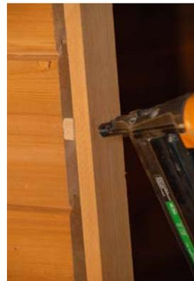
Step 7: Once the hinge side is mounted. Close the door and adjust the rest of the jamb into the right position. Shims will be required, use a brad nailer to lock in the jamb/shims. A door should have at least 4 shim locations on the side and 2 on the top.
