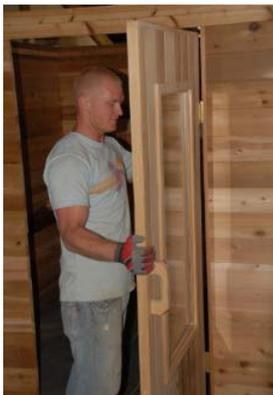
Step 5: Put pre-hung door in place. Be sure to center the door/ door jamb on
