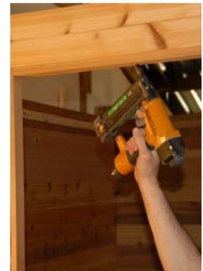
NOTE: Once the door jamb is set to the to the right location and showing the desired reveal, you can use set screws in the jamb or secure with brad nails. Finish out the door frame with the pre-cut door trim (door casing) using the brad nailer.
