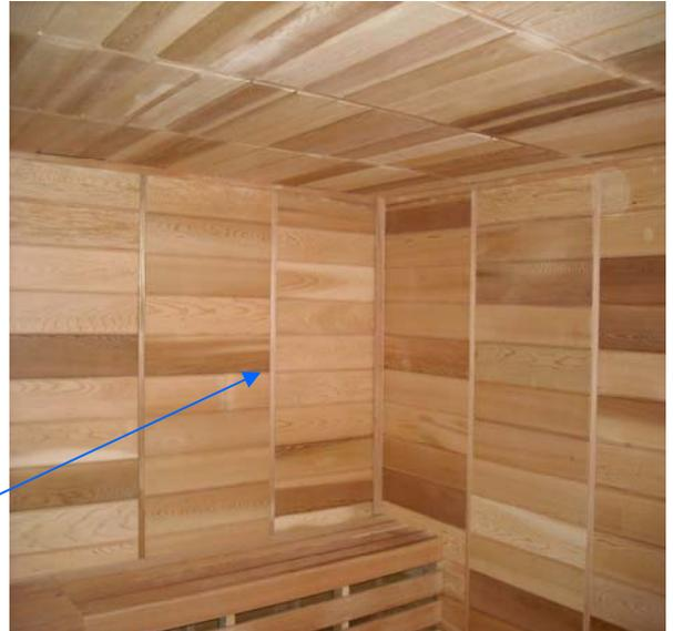
Step 4: Once all of the wall panels are all in place you will install the wall trim. Start with the 1" vertical trim in between the wall panels attaching the trim with 1 1/2" brad nails.
