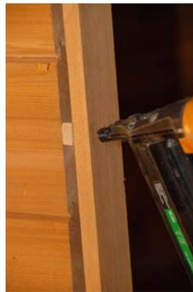
Step 8: Once the hinge side is mounted. Close the door and adjust the rest of the jamb into the right position. Shims will be required, use a brad nailer to lock in the jamb/shims. A door should have at least 4 shim locations on the side and 2
