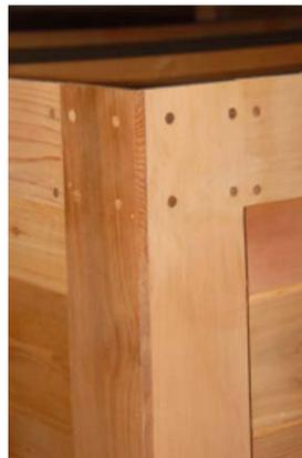
Step 11: All interior and exterior trim pieces are labeled and ready for mounting. They can be brad nailed into place. The exterior trim can be fastened with supplied screws on the corners (as shown above). Plug the holes with the supplied cedar dowels for a beautiful finished look
