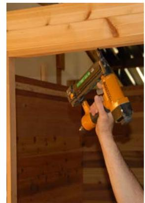
NOTE: Once the door jamb is set to the to the right location and showing the desired reveal, you can use set screws in the jamb or secure with brad nails. Finish out the door frame with the pre-cut door trim (door casing) using the brad nailer.
