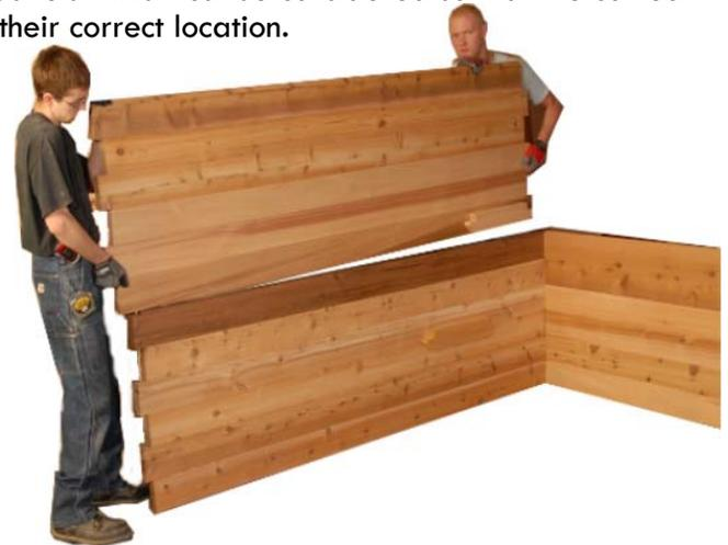
Step 3: Place the lower front wall panels in place after all three "middle-wall" panels are in place. Be sure all joints are screwed tightly at this point.
