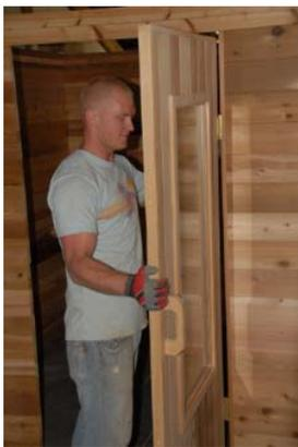
Step 6: Put pre-hung door in place. Be sure to center the door/door jamb on the wall.
